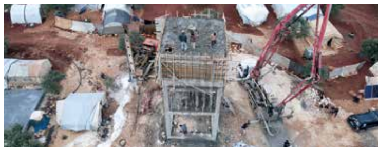
Water tower during construction
