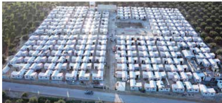
The same camp after infrastructure and construction was completed.
