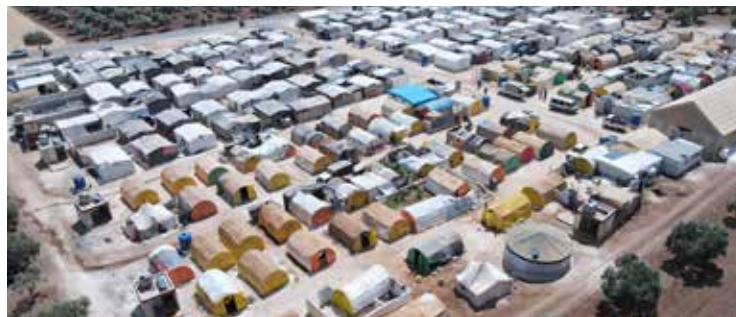
One of the three camps transformed by the Dignified Shelter Project before construction.
